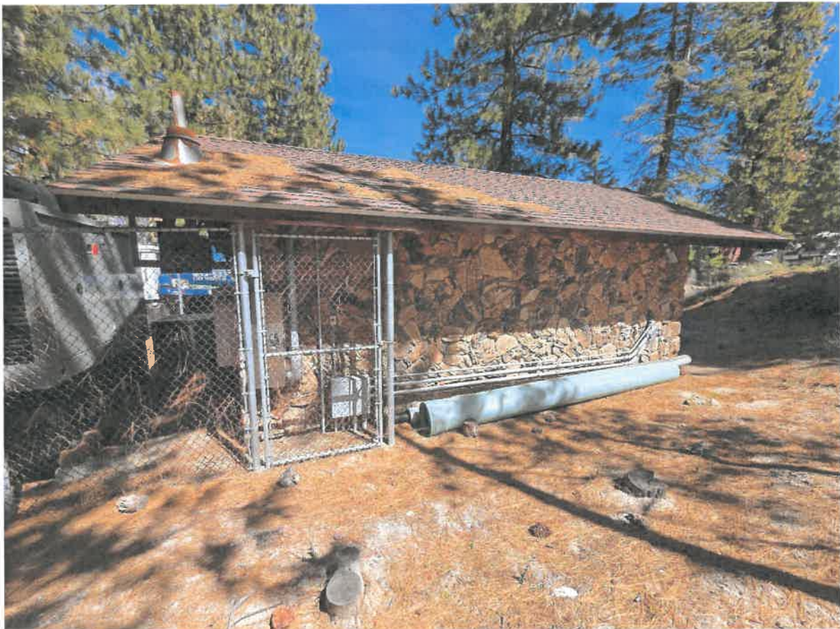
Market Street Lift Station
