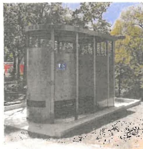
One of the Portland Loo facilities that Truckee Meadows Water Authority installed at a local park in Reno, Nev.
